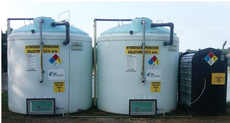
Sampling of the lagoon by USP Applications Specialists demonstrated that within 24 hours, the hydrogen peroxide addition to the aerated lagoons resulted in measurable increases in DO and elimination of H<sub>2</sub>S odors. With continued dosing of hydrogen peroxide, the DO levels increased incrementally over the next several days. By the
